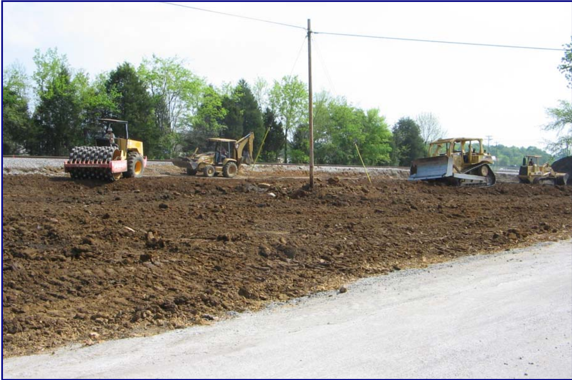
April 18, 2006 – Grading at Martha Station
